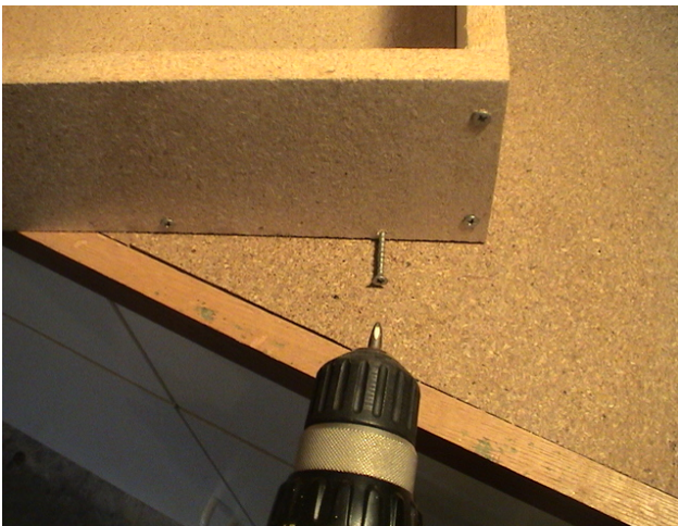
Assembling the form
