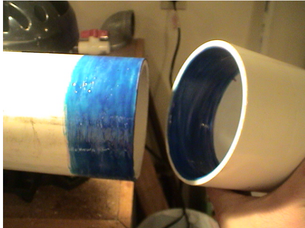
Pipe and Coupling with PVC Cement
