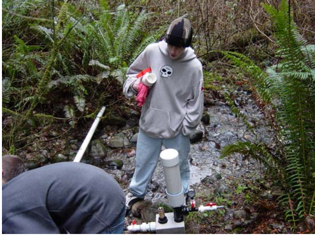
Hooking up the drive pipe.
