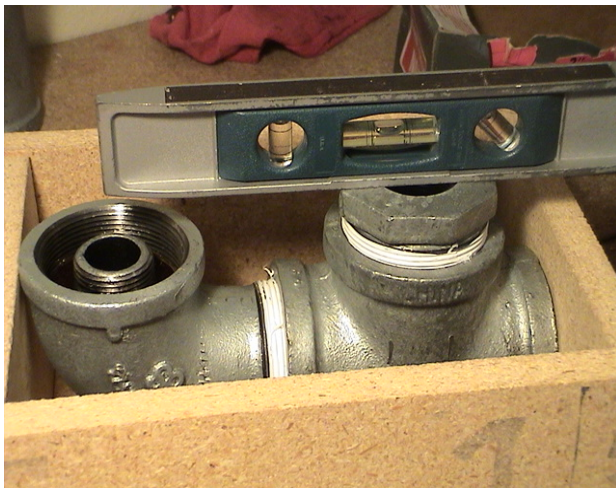
Leveling the HRP1-1 in the form
