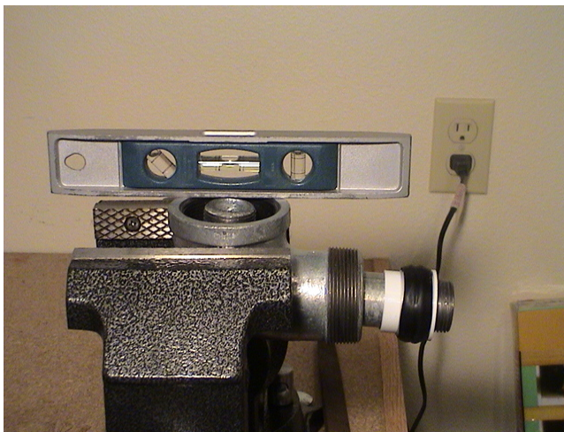
Leveling the 2" Street Elbow
