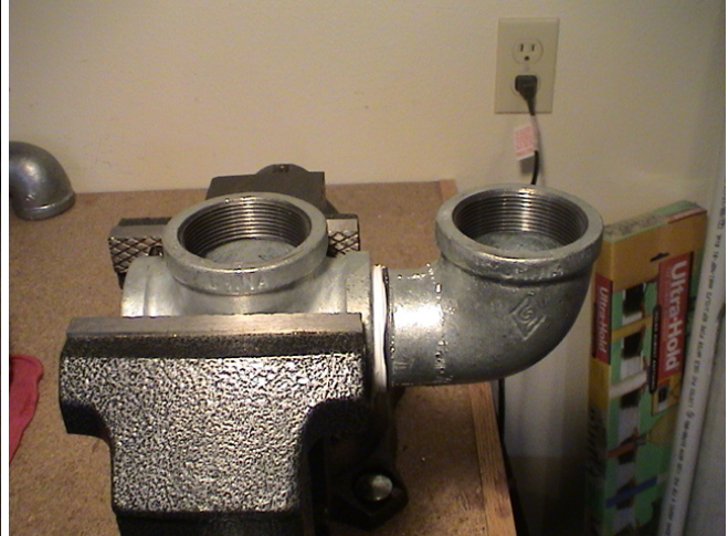
The 2" Street El installed
