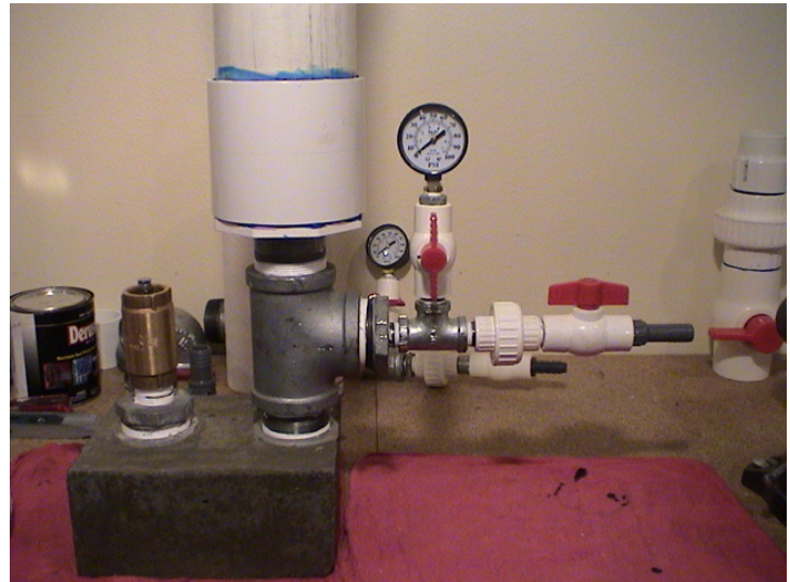
Adding ball valves, gauge and union
