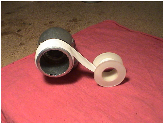
Wrap the Teflon tape clockwise
