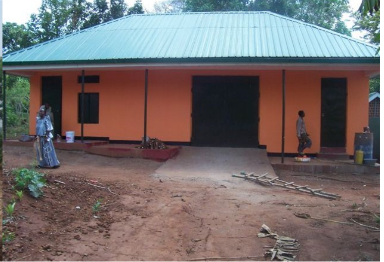
Storage Shop and Caretaker Housing, Nabisooto 2011
