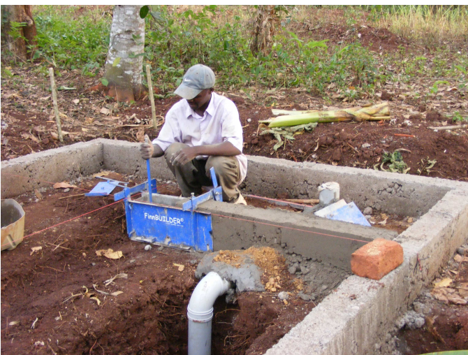
Doc working on the bathroom.
